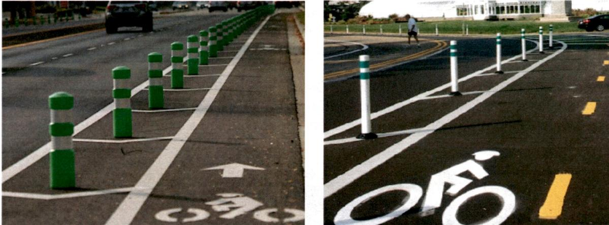
**Figure 7 – K71 (green 12-inch bollard) and standard 2-inch white delineator**
