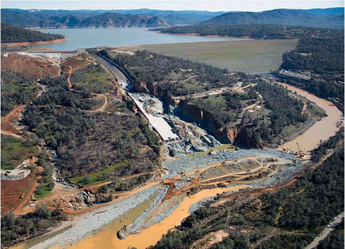
**Figure 13-5. Oroville Dam Emergency Spillway Failure in Spring 2017**
